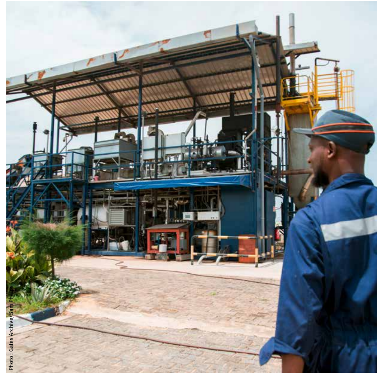
The Janicki Omni Processor was installed in Dakar, Senegal, in 2015 and now treats the faecal sludge of up to a hundred thousand people.
