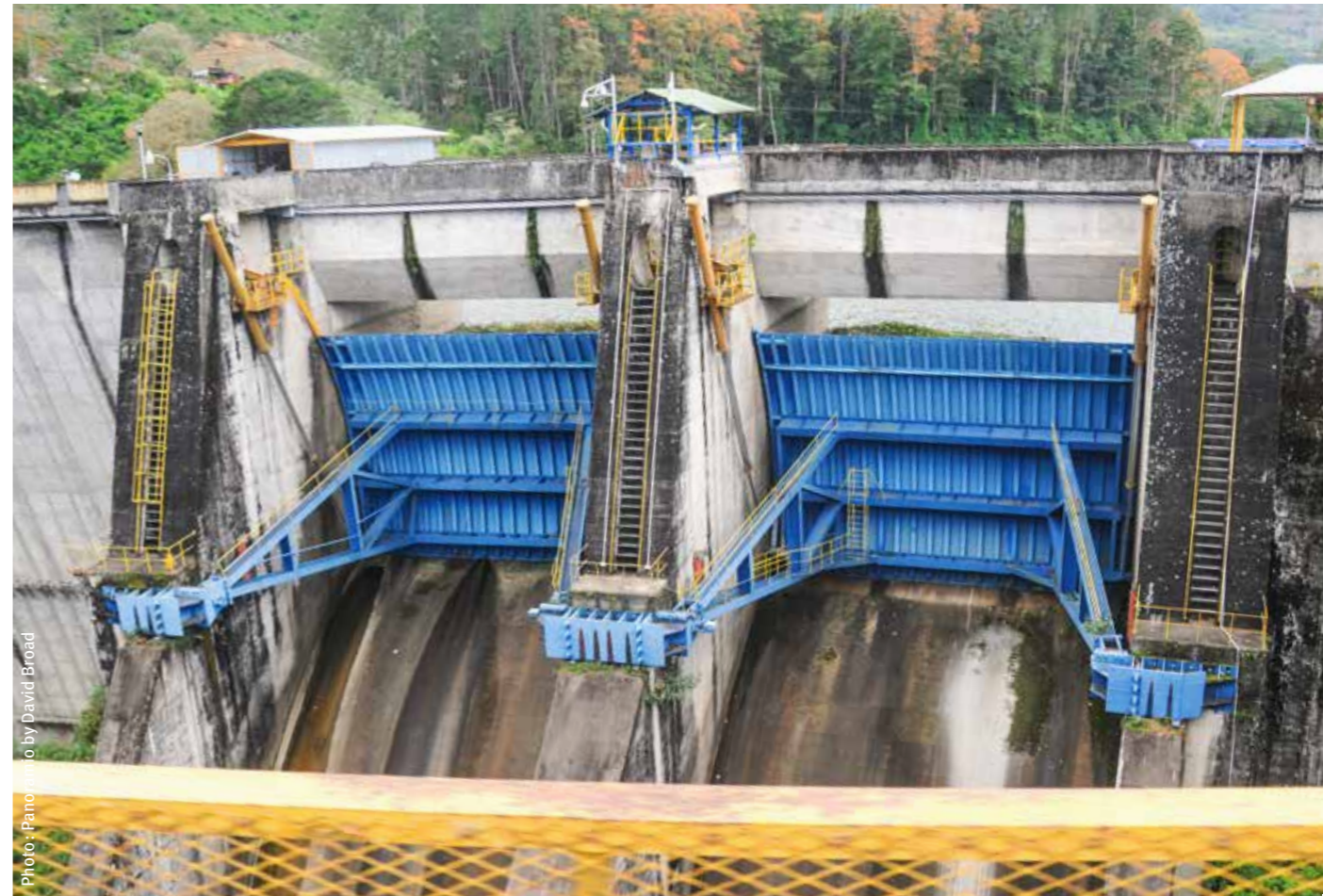
The Cachi hydroelectric plant now has capacity to generate almost 160 MW after expansion works were carried out.
